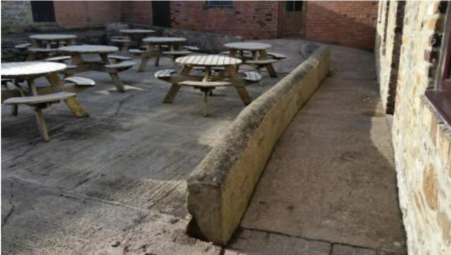
Tea Room Courtyard 2
