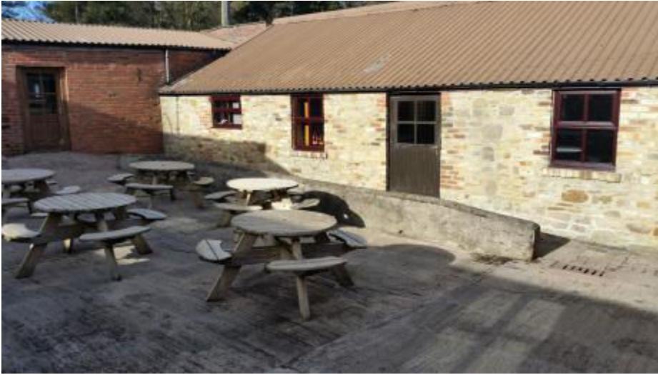
Tea Room Courtyard 1
