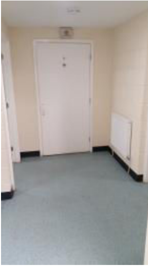
Disabled Toilet - External
