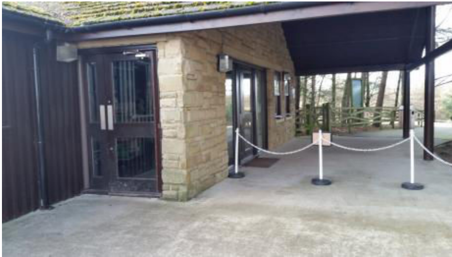
Entrance / Exit Door
